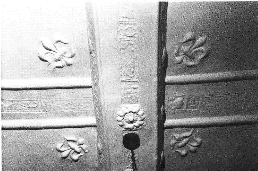
Brick House Farm, Hitcham: detail of the plaster ceiling in the parlour.
